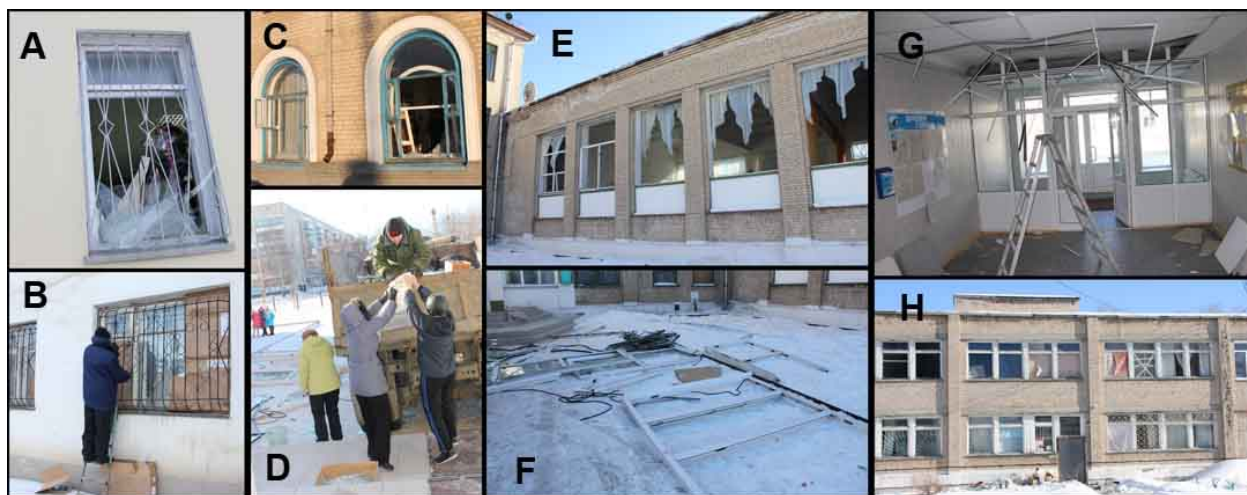
Fig S36. Examples of glass damage in pictures from Yemanzhelinsk. (A) Broken window glass. (B) Initial protection against wind. (C) Window frames blown in. (D) Clean up. (E) , (F) and (H) Lost window frames in school. (G) Suspended ceiling sucked down. Photos by Victor I. Gubar of Yemanzhelinsk.
